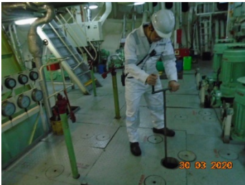
Opening VALVE for F.O transfer
